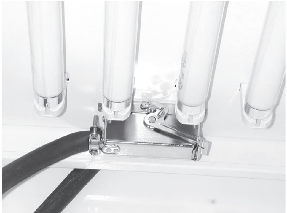
*Proper Installation of Shelf Lamp Connection*
